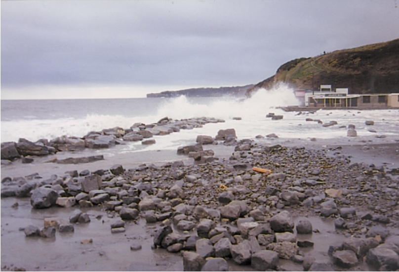
Fig. 3. Storm overwash, Colhuw Beach February 1990.
