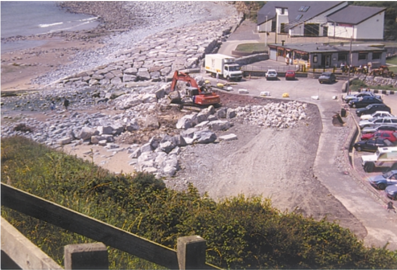
Fig. 7. Remedial reconstruction undertaken at Colhuw in the summer of 1998.
