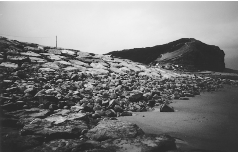
Fig. 4. Beach side view of the Colhuw revetment.
