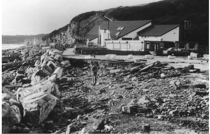
Fig. 5. View westwards at Colhuw showing the November 1996 storm damage.
