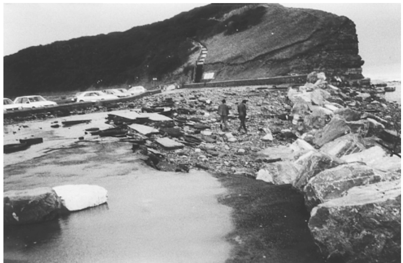
Fig. 6. View eastwards at Colhuw showing the November 1996 storm damage.
